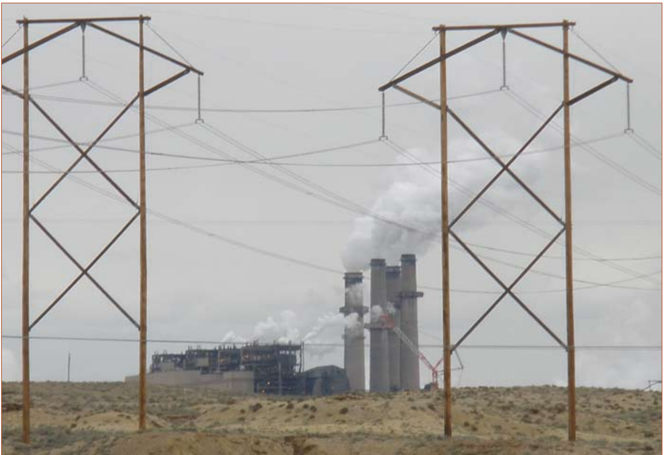
San Juan Generating Station near Farmington, New Mexico.
