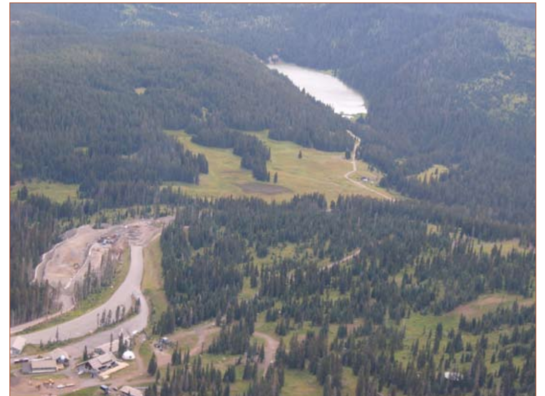
The Village at Wolf Creek is planned for the alpine meadow between Alberta Reservoir and the existing Wolf Creek Ski Area parking lot, as seen in this aerial photo.
