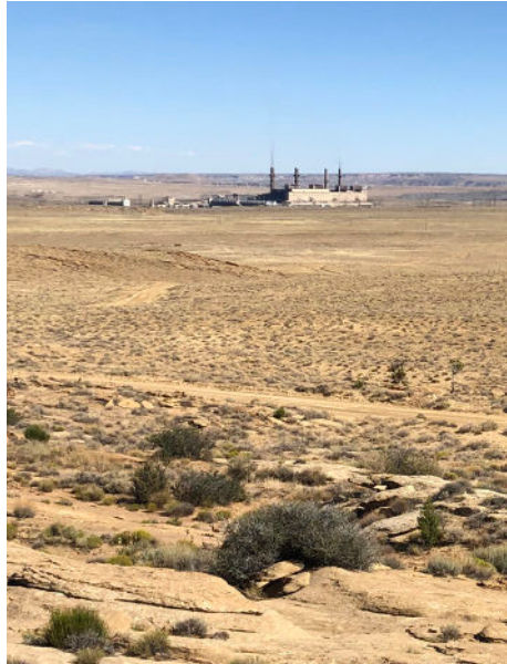
San Juan Generating Station, and the site of the planned Shiprock Solar Project.
